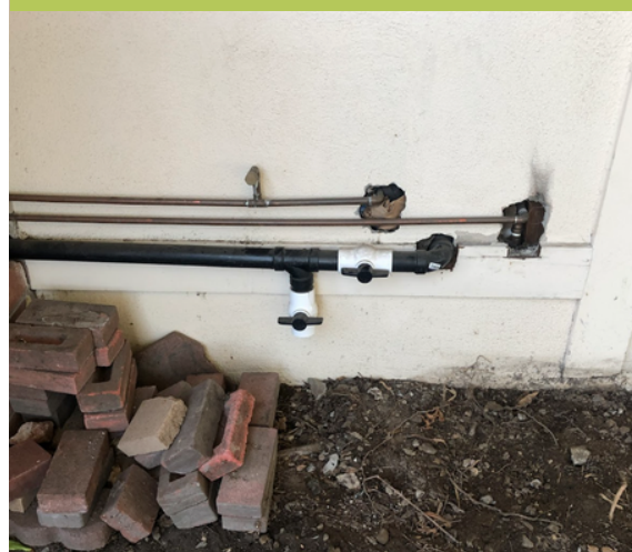
Simple greywater system that drains water from the clothes washer directly to the landscape.
