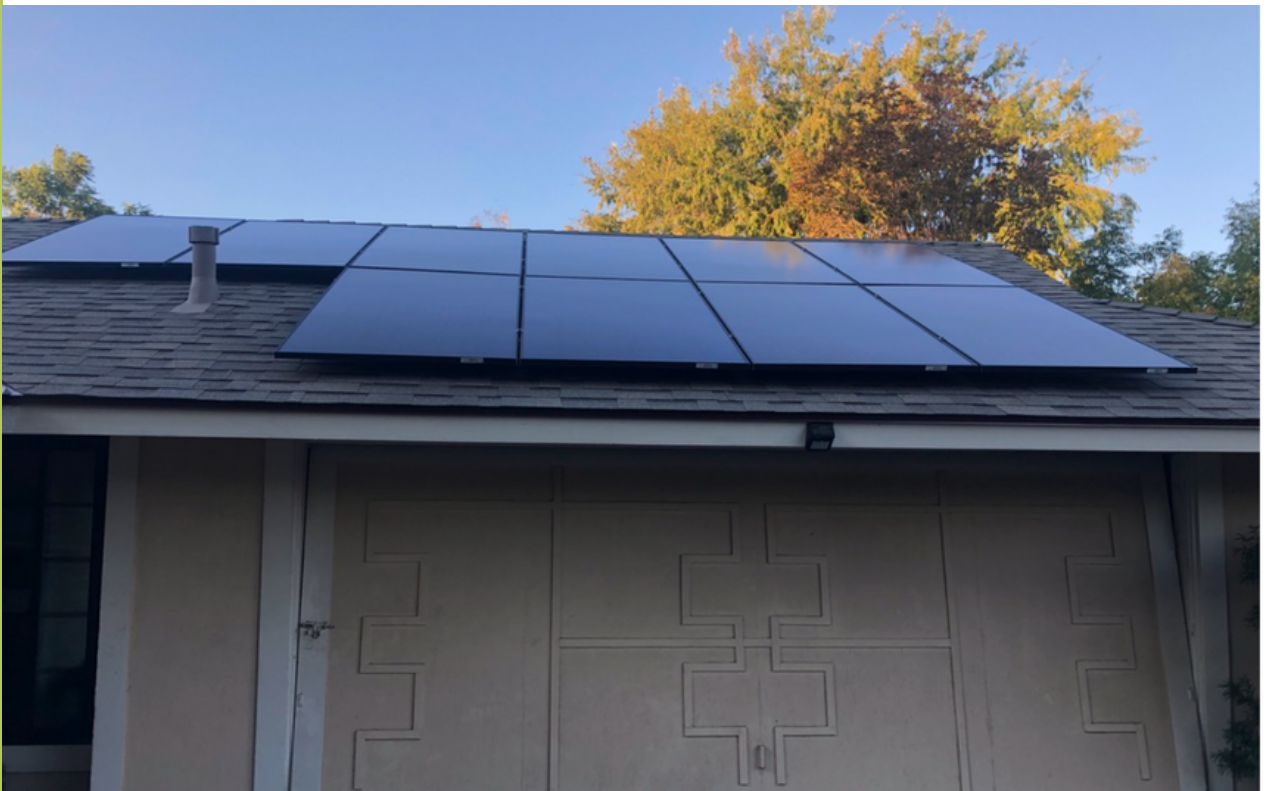
Solar panels and an EV charger from HPM Solar .
